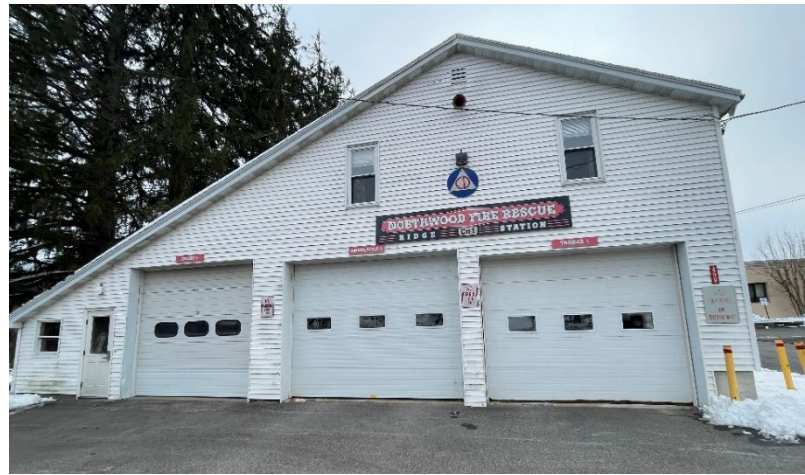
Ridge Fire Substation
