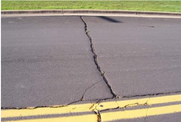
Transverse Crack
