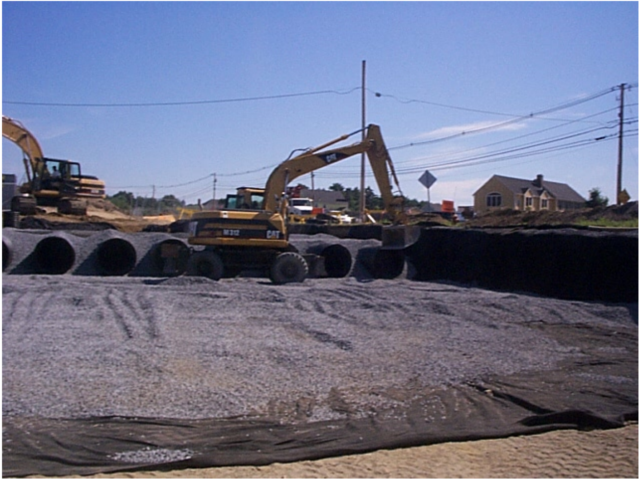
Large subsurface infiltration system under construction.
