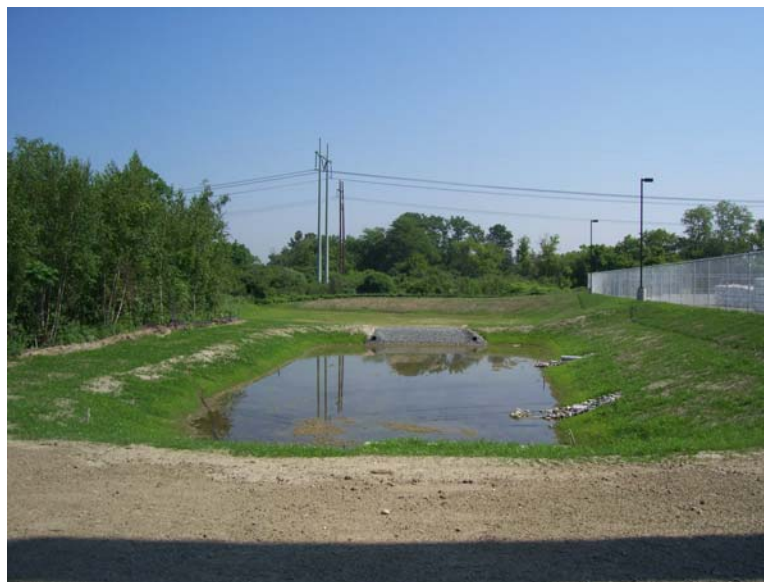
Small Detention Pond at an Industrial Facility
